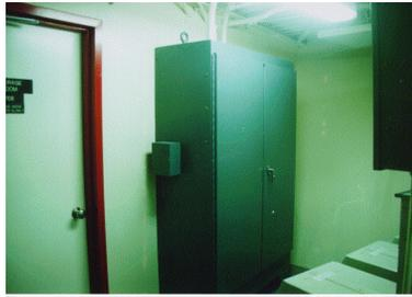
Figure 1.10: *This big box in the UPS/Electrical Room (see Figure 1.2) houses the dome motor controllers, which power the four motors that rotate the dome.*
