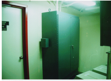
Figure 1.10: This big box in the UPS/Electrical Room (see Figure 1.2) houses the dome motor controllers, which power the four motors that rotate the dome.
