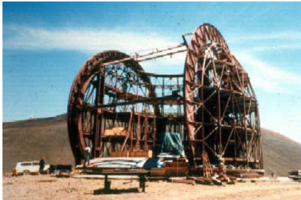
Figure 3. Assembly of the dome on Mauna Kea. Here the shutter doors are being assembled on the tracks "in situ".
