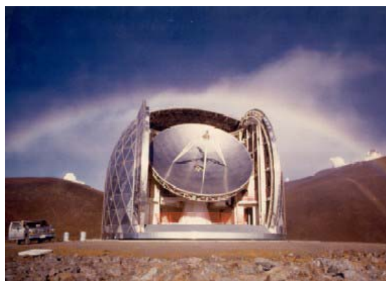
Figure 8. The completed observatory. The dome azimuth drive is slaved to follow the telescope which allows internal room for control and receiver and detector functions. At any given time the CSO supports 5 heterodyne receivers (Cass and left Naysmyth), 2 cameras (Bolocam – Cass), (SHARC II–right Naysmyth), and the grating–(right Naysmyth).
