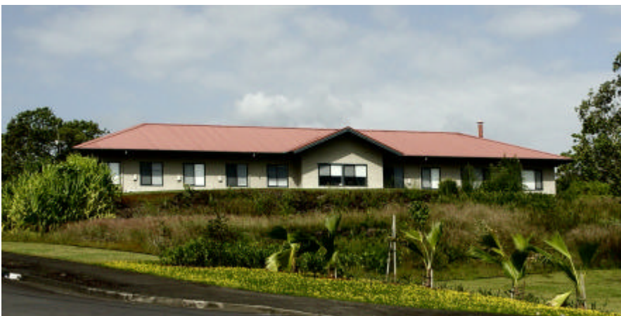
The eastern face of the new Gimble Building
