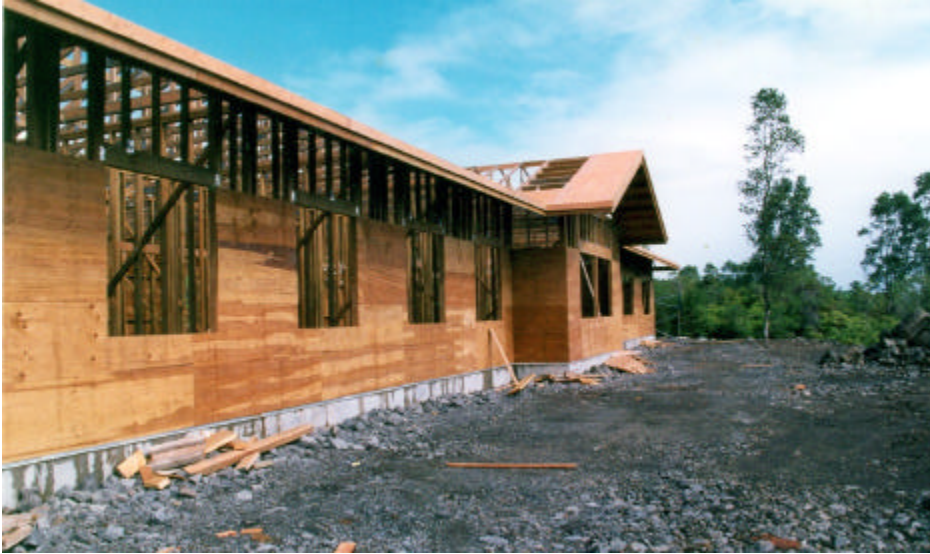
The east-facing façade. Each window will be a separate office.
