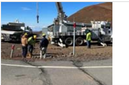
HELCO prepping and making precautions.
