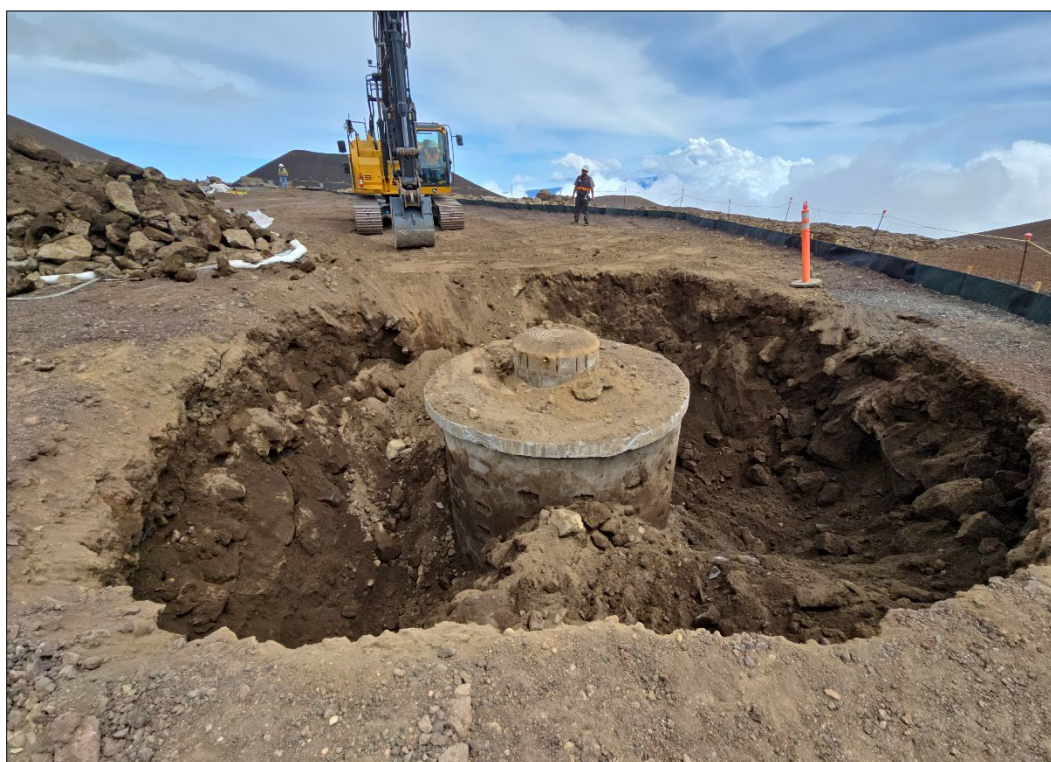
Figure 17. Deere 245P excavating out the existing cesspool, view to the south.
