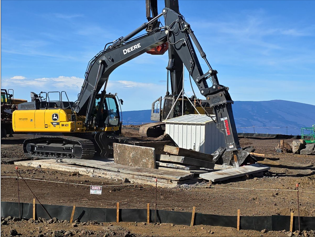
Figure 14. Deere 350P with a hydraulic hammer attachment hoe ramming the concrete foundation of the water pump shed, view to the south.
