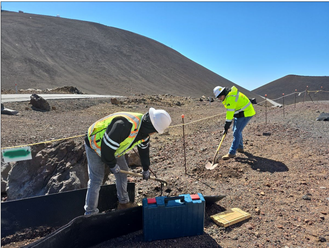
Figure 9. Silt erosion fencing around the perimeter of the observatory, view to the southeast.
