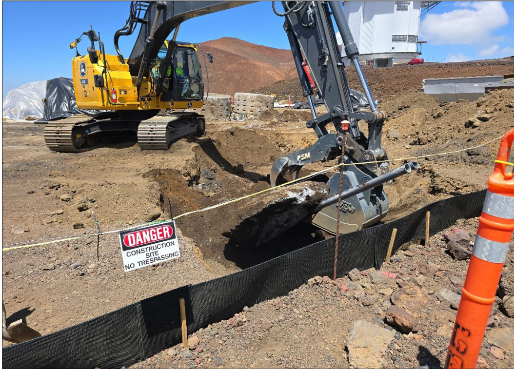
Figure 20. Deere 245P with a 32-inch bucket removing the electrical conduit concrete pad, view to the southwest.
