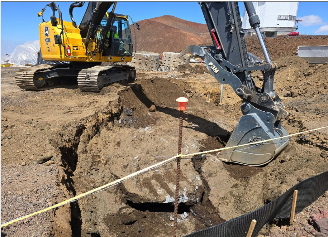
Figure 19. Deere 245P with a 32-inch bucket removing the electrical conduit concrete pad, view to the southwest.
