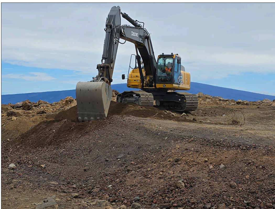
Figure 27. Deere 350P with a 60-inch bucket grading of the project area, view to the south.
