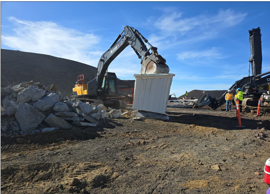
Figure 15. Volvo 350 with a 60-inch bucket removing the water pump shed, view to the southeast.
