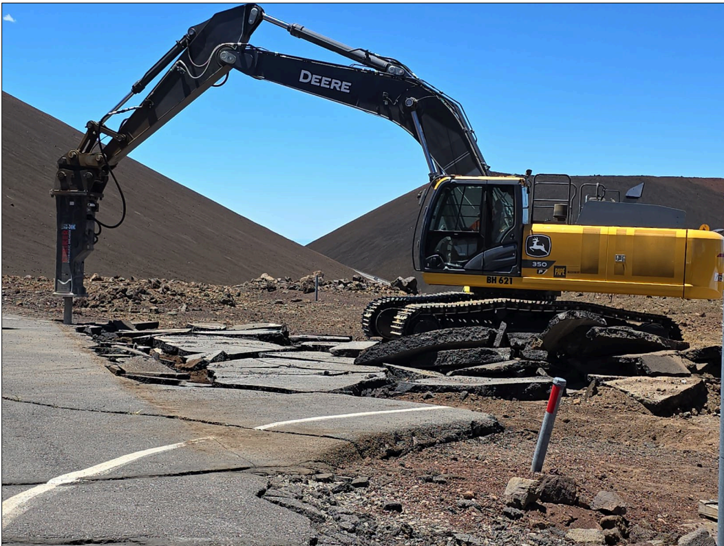
Figure 31. Deere 350P with hydraulic hammer attachment to remove the existing asphaltic driveway entrance, view to the south.
