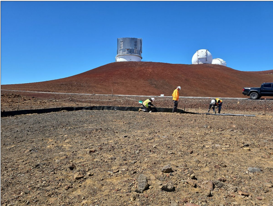
Figure 11. Silt erosion fencing around the perimeter of the observatory, view to the north.
