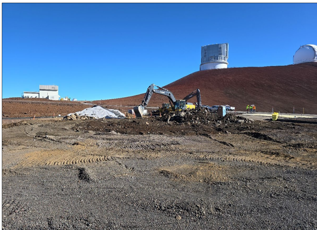
Figure 13. Post-hoe ramming of the concrete foundation of the observatory, view to the north.
