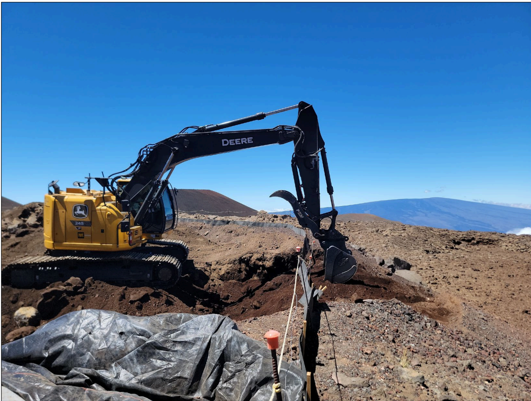
Figure 25. Deere 245P with a 32-inch bucket grading of the project area, view to the southwest.
