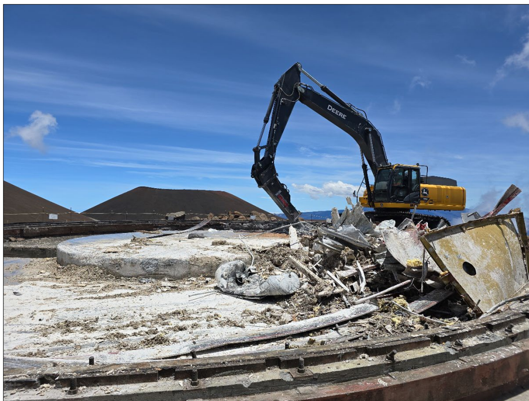
Figure 12. Deere 350P with a hydraulic hammer attachment hoe ramming the concrete ring foundation of the observatory, view to the south.
