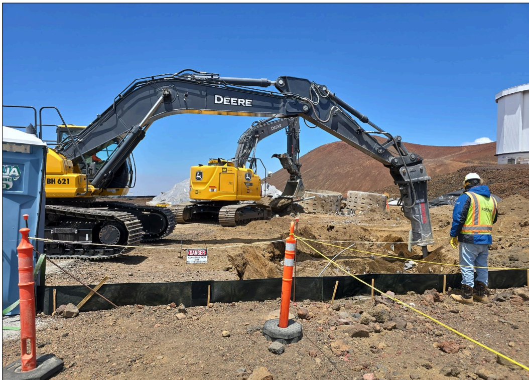
Figure 21. Deere 245P with a hydraulic hammer attachment to remove more of the electrical conduit concrete pad, view to the southwest.
