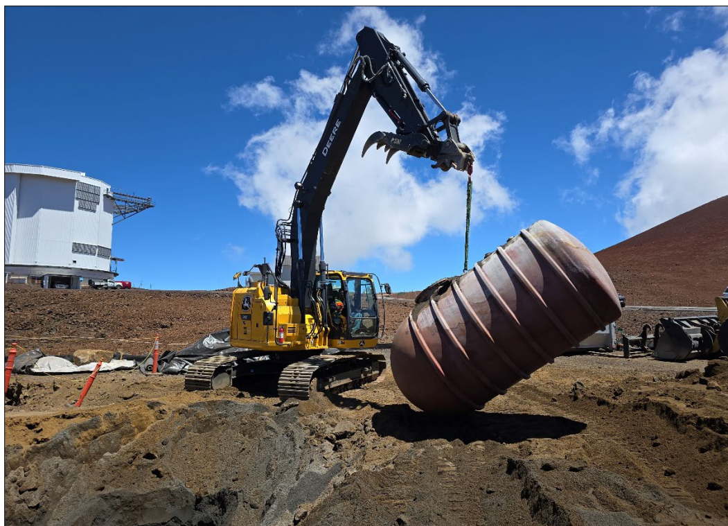
Figure 16. Deere 245P removing the 2,000-gallon water tank, view to the west.
