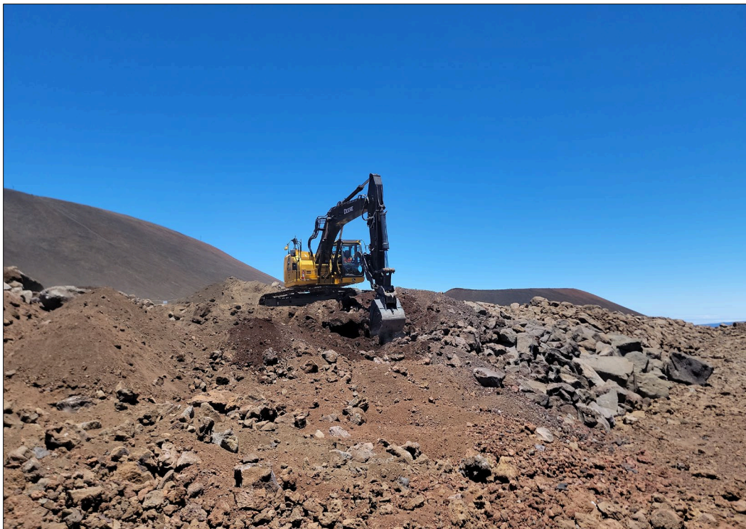
Figure 26. Deere 350P with a 60-inch bucket grading of the project area, view to the southeast.
